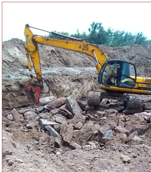
Works at the new dam
